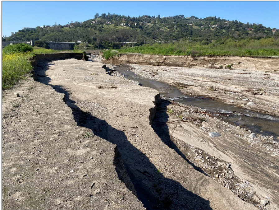
Photo 6. View of middle section of the sediment removal area, facing southwest
