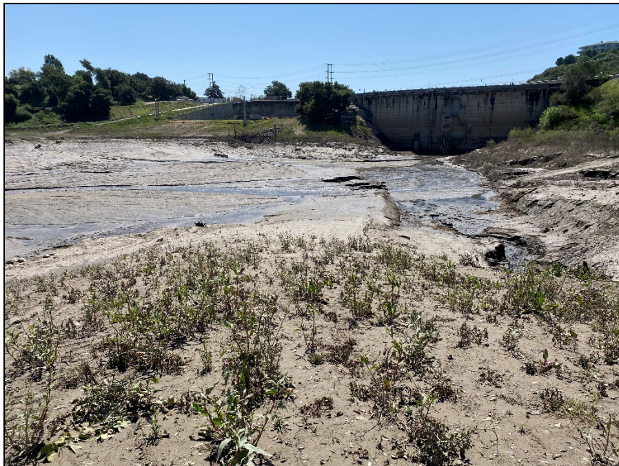
Photo 2. View of initial sediment removal area, facing southeast.
